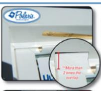
All Polaris replacement windows have separate extrusions for the head of the window. This provides twice as much overlap when closed, preventing air infiltration, and a much cleaner look from inside the home.
